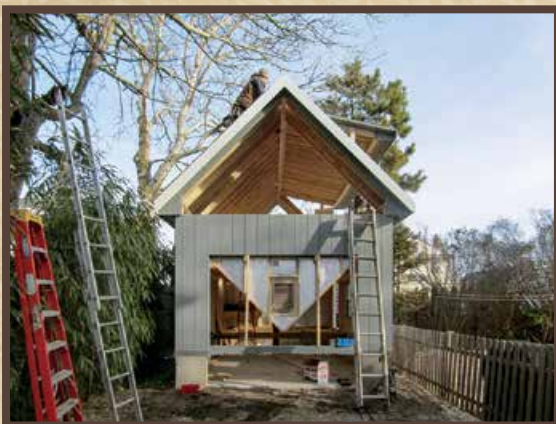
Hinge Roof Under Construction
