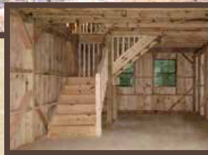
Rough Cut Oak Framing
