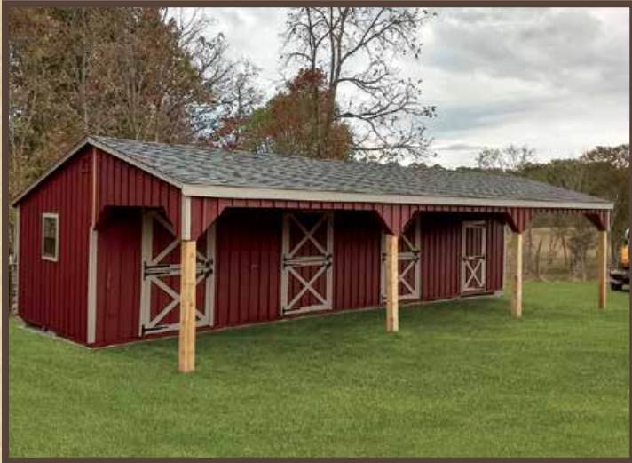
(521) 12x40 Horse Barn 3 Stalls and Tack Room • 10x40' Lean To • 1x10 Pine Board and Batten Siding: Barn Red • Trim: Clay • Roof: Charcoal
