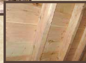
3x6 Rough Cut Hemlock Rafters @ 24" O.C. with 1x10 Pine Ship Lap Roof Sheathing or 1x8 Pine Tongue and Groove
