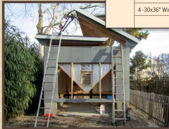
Jacking up Roof
