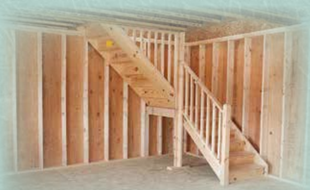
First floor with stairs
