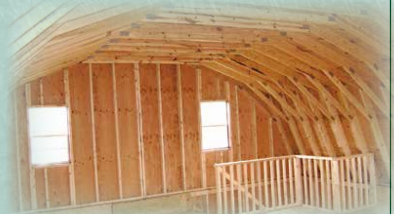
Plenty of second floor headroom
