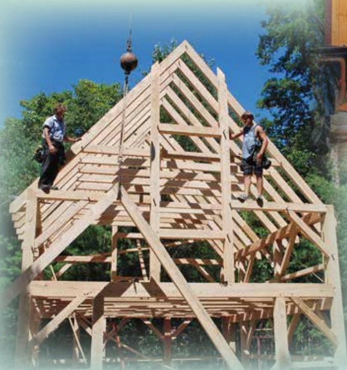
Mortise and tenon framing
